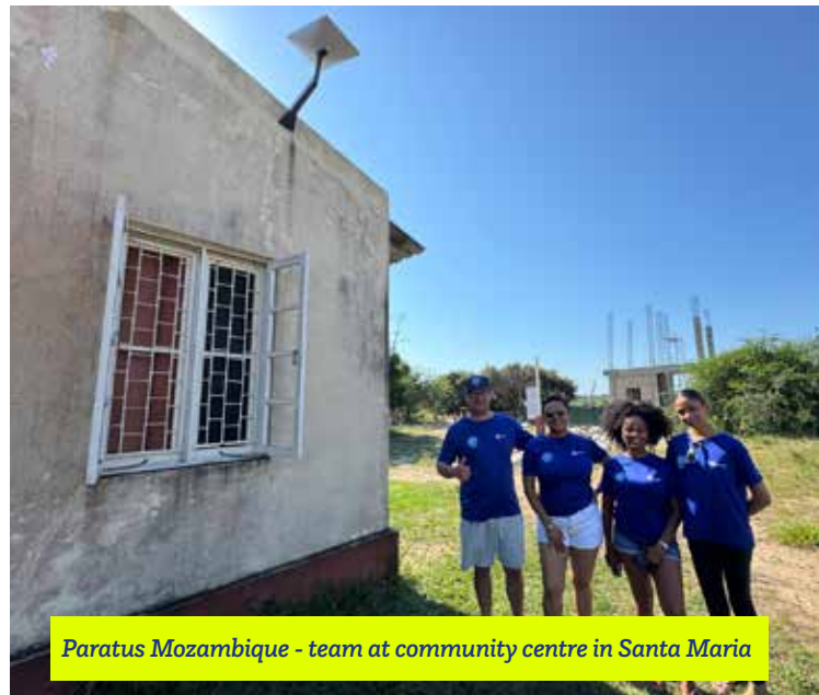
Paratus technicians installing fiber
